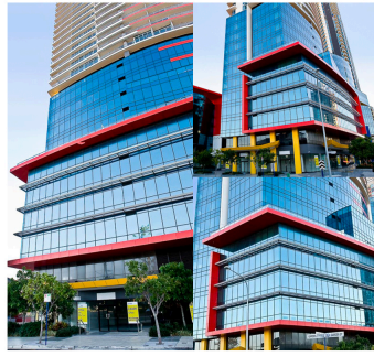
AGC Glass, AU 2017 Began extreme ocean front salt spray. Invisible Shield was used to treat glass for long term protection against contaminants and permanent corrosion.
